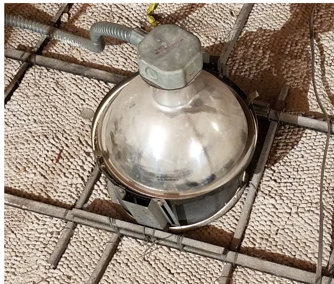
EXISTING DOWNLIGHT WITH REFLECTOR INSTALLED ON HOUSING FLANGE
