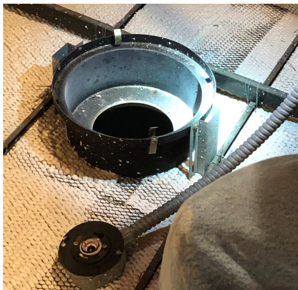
EXISTING DOWNLIGHT HOUSING WITH REFLECTOR REMOVED
